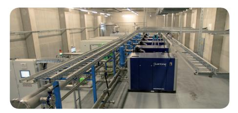
CompAir was responsible for storage, water cooling with pumps and heat exchangers, and all of the pipework.
