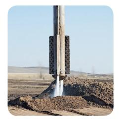
With the help of water and compressed air the vibrator works its way up to a depth of 60 metres.
